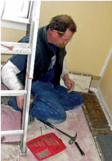
Inside the tower, tight space proved challenging for the work team to negotiate.
